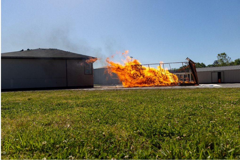
Figure B3.1. Photograph of wind-driven flame spread testing at the IBHS Research Center in Richburg, South Carolina.
