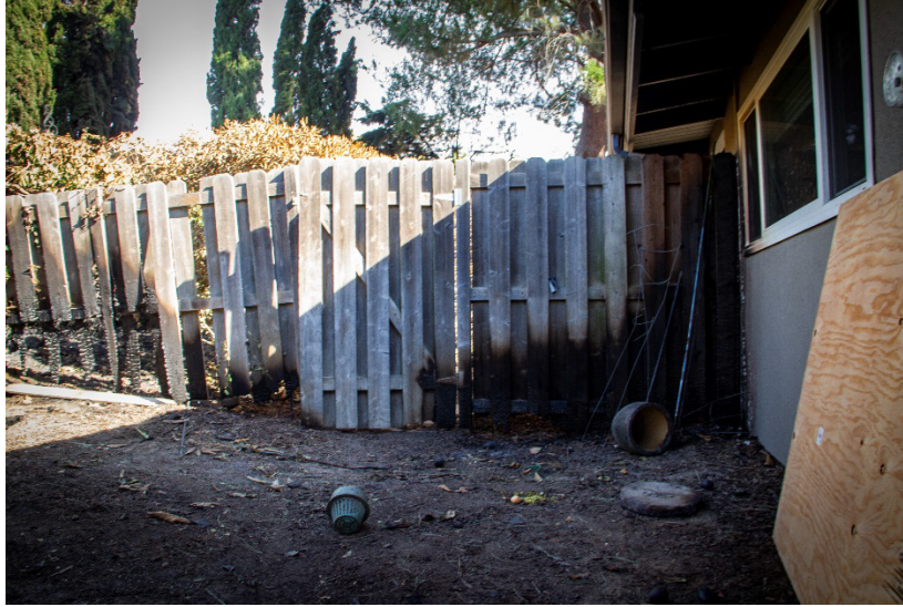
Figure B4.2. Photograph of a fence, following the 2024 Mountain Fire in Camarillo, CA, which had ignited adjacent to a home where fire spread to the wall of the structure. In this case fire service intervention and the presence of noncombustible wall cladding (stucco) helped avoid ignition of the structure. The window frame on the right side of the image was damaged, and there was evidence of sufficient radiant heat to damage the paint in the eaves of this home. Photograph by Evan Sluder.
