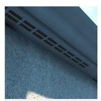
Because of their geometry, radiant heat can build up in an open eave and ignite exposed materials. Flames from nearby fuels such as a shed or vegetation can also ignite eaves.
